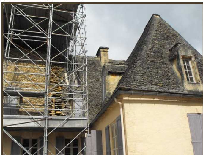
REPAIRS TO THE STONE ROOF
